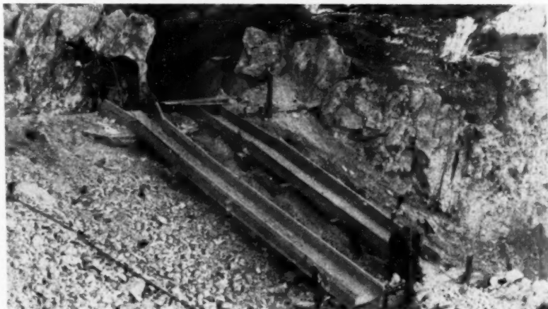
The mule, Beryl, stands near the tunnel entrance. High-grade beryl is dumped down wooden chutes then cobbled and sorted while being stacked on a platform.
